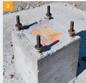
3 Remove the PPL template and level the nuts.
