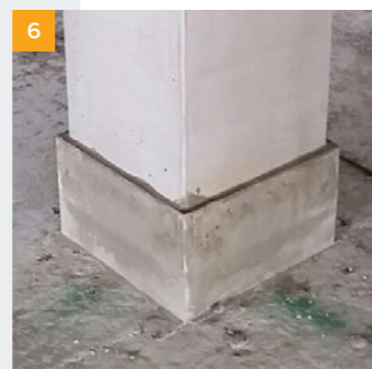
6 Grout the joint and the column pockets.
