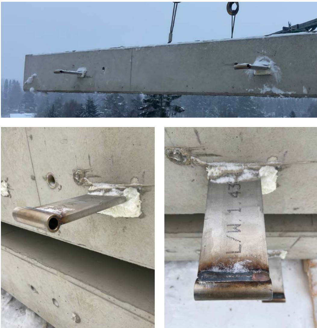
Figure 16. Balcony slab with PS Part B.
