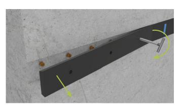
7. After removing the Rebate Former Board, the Connector Plugs are visible. Screw them off using the Plug Release Key (see Annex B - Accessories). Connector Plugs can be removed just before assembling Threaded Bars.
