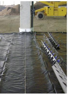
3. The joint can then be fixed in position using pins. Fixing pins should be 14 mm – 16 mm diameter and at least 300 mm longer than the joint height. A good practice is to use 14 x 600 mm fixing pins.
