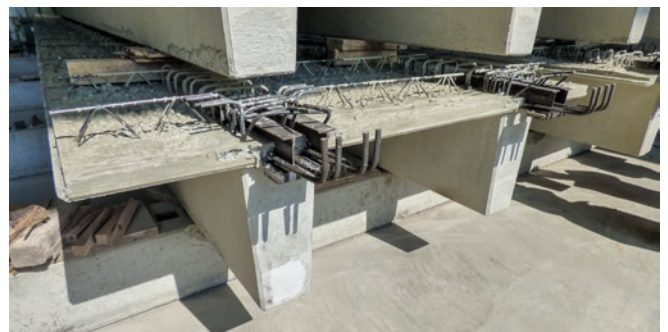
Figure 11: TT slabs equipped with TWIN Corbel
