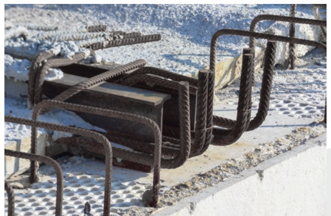
Figure 13: Assembled TT slab with TWIN Corbel
