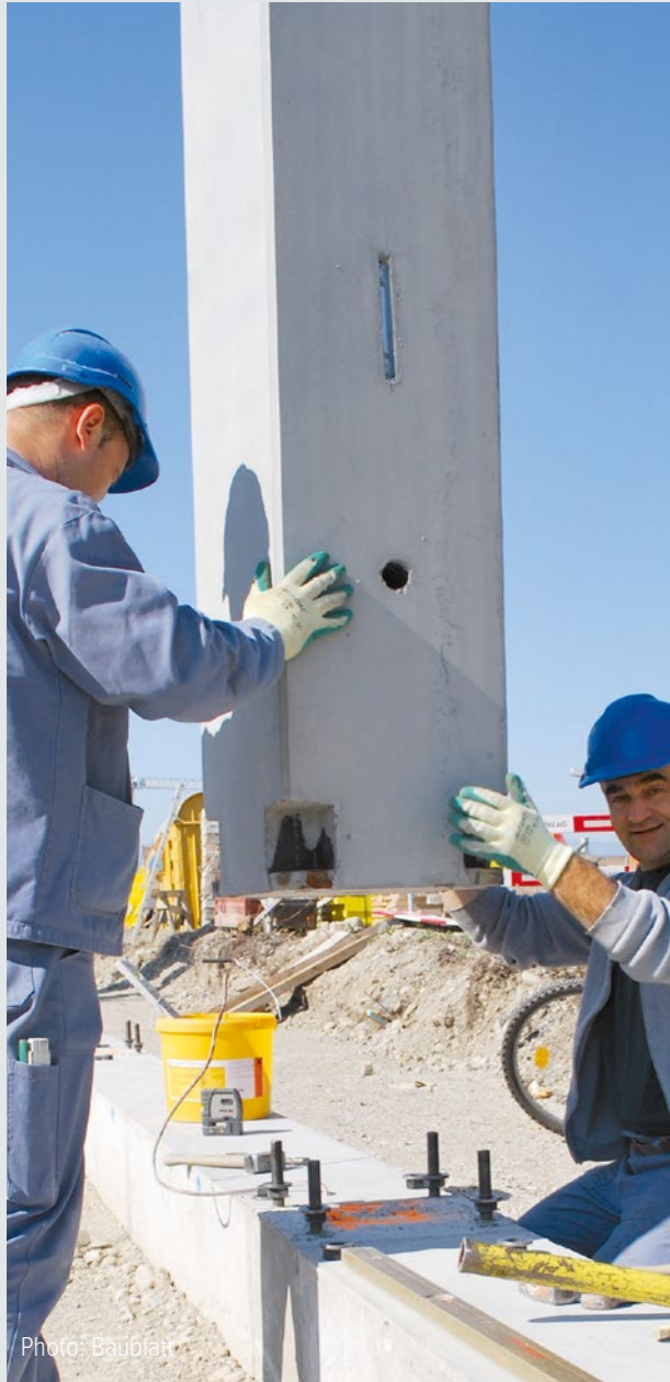
Photos showing the steps in the process of assembling the Peikko Column Shoes.
