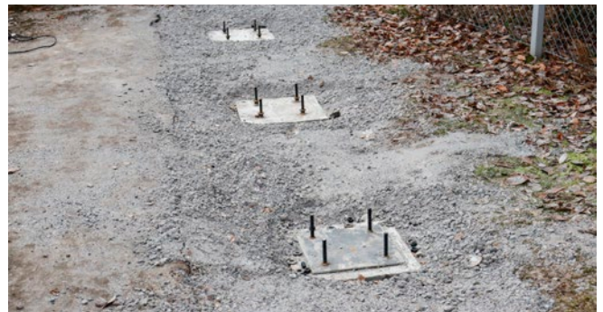
FIGURE 4. CASTED FOUNDATION BLOCKS INSIDE THE GROUND
