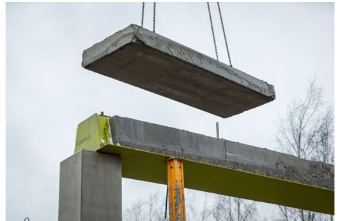
FIGURE 11. ASSEMBLED PRECAST FRAME
