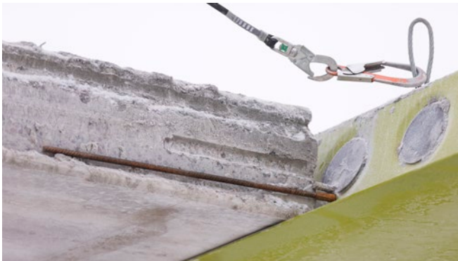
FIGURE 20. REASSEMBLY OF HC SLAB UNITS ON DELTABEAM® GREEN, "WET" JOINT ON THE LEFT AND "DRY" ONE ON THE RIGHT
