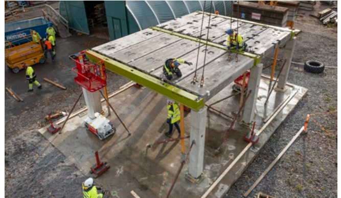
FIGURE 11. ASSEMBLED PRECAST FRAME
