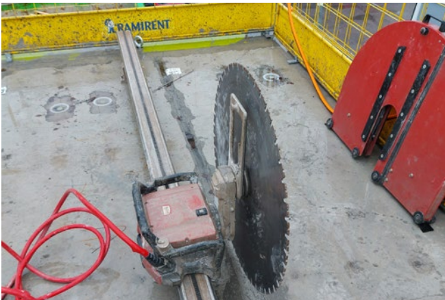
FIGURE 12. DISASSEMBLY OF GROUTED SLAB JOINTS AND REMOVAL OF HC SLAB UNIT
