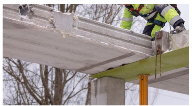
FIGURE 20. REASSEMBLY OF HC SLAB UNITS ON DELTABEAM® GREEN, "WET" JOINT ON THE LEFT AND "DRY" ONE ON THE RIGHT
