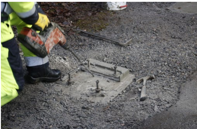
FIGURE 7. REMOVAL OF GROUT PAD WITHOUT RELEASE AGENT
