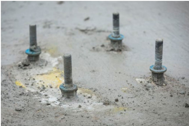
FIGURE 17. CLEANED FOUNDATION READY FOR REASSEMBLY OF PRECAST COLUMN
