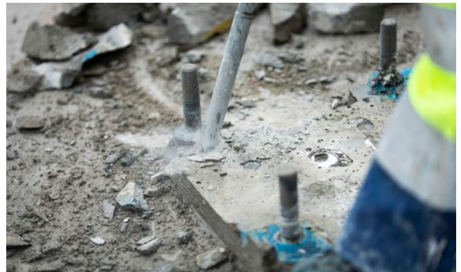
FIGURE 16. REMOVING THE GROUT PAD
