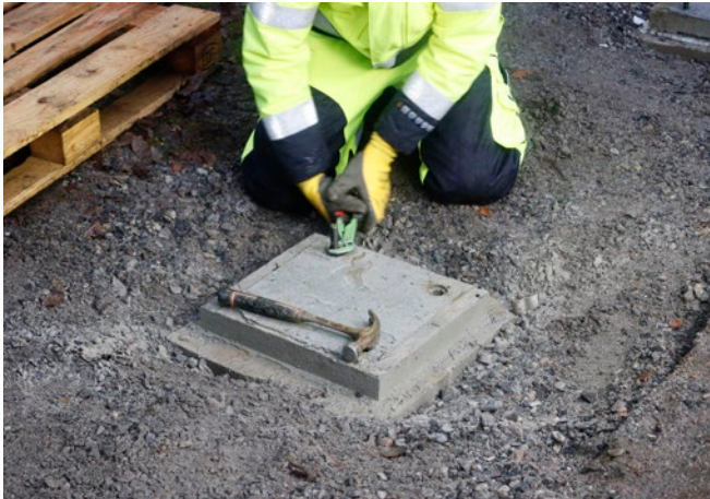
FIGURE 6. REMOVING THE THREADED BARS FROM ANCHORING COUPLERS
