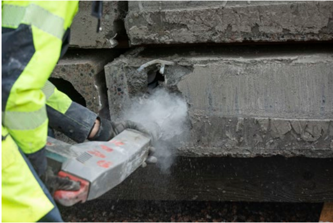
FIGURE 18. CLEANING PROCESS OF VOID AND CLEANED VOID OF HC SLAB UNIT
