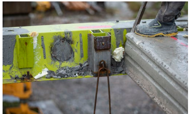
FIGURE 13. REMOVING OF CONCRETE BY USING A CHIPPING HAMMER
