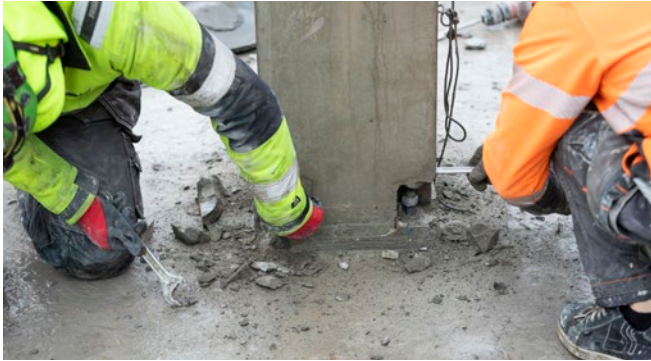
FIGURE 15. OPENING THE NUTS
