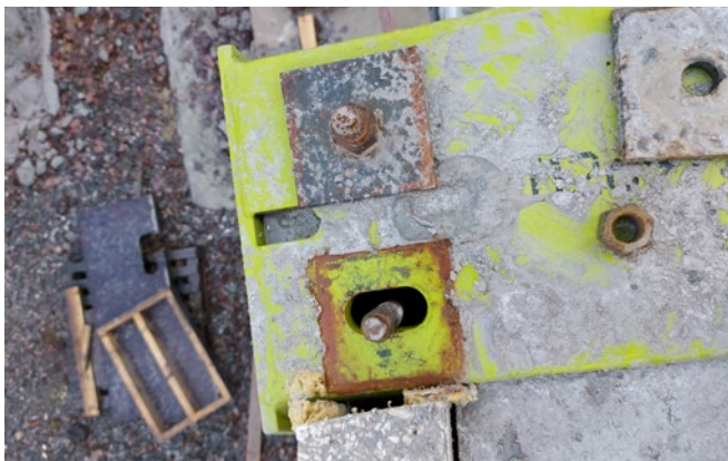
FIGURE 14. DISASSEMBLY OF DELTABEAM® GREEN COMPOSITE BEAMS
