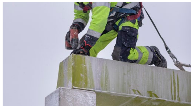
FIGURE 20. REASSEMBLY OF HC SLAB UNITS ON DELTABEAM® GREEN, "WET" JOINT ON THE LEFT AND "DRY" ONE ON THE RIGHT
