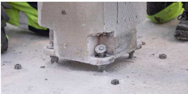
FIGURE 19. REASSEMBLY OF PRECAST COLUMNS ON THE FOUNDATION SLAB
