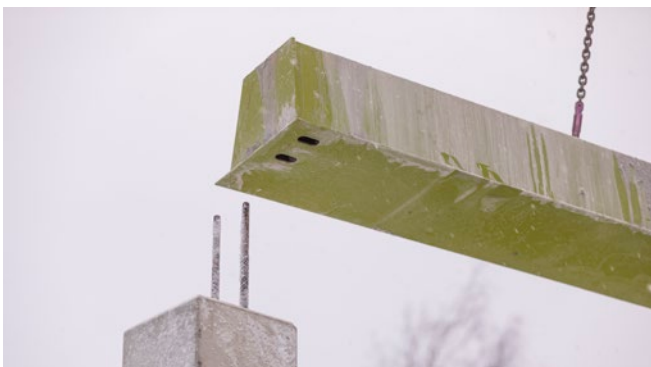
FIGURE 21. REASSEMBLY OF DELTABEAM® GREEN COMPOSITE BEAMS ON PRECAST COLUMNS
