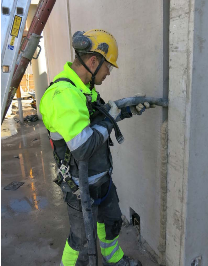
Figure 23. Casting of the joint.
