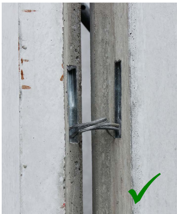
Figure 22. Correct installation of wire loops.
