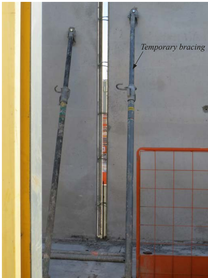
Figure 19. Precast wall installed at final position and secured by temporary bracing.
