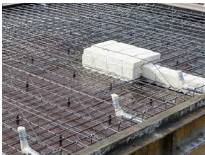
Figure 20. PD ties after installation of insulation.
