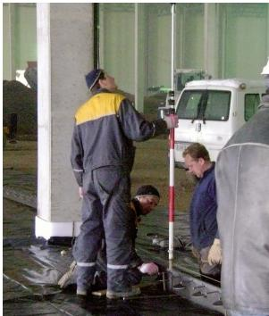
3. The joint can then be fixed in position using pins. Fixing pins should be 14 mm - 16 mm diameter and at least 300 mm longer than the joint height. A good practice is to use 14  $\times$  600 mm fixing pins.
