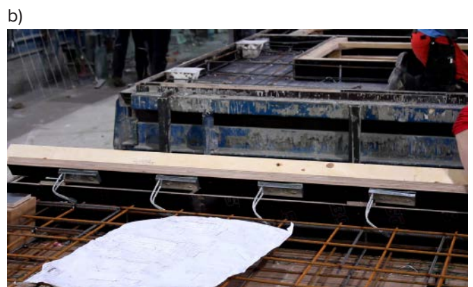
Figure 15. Installation of the PVL® Connecting Loop to wooden formwork: a) directly to side of formwork; b) to the wooden recess channel.
