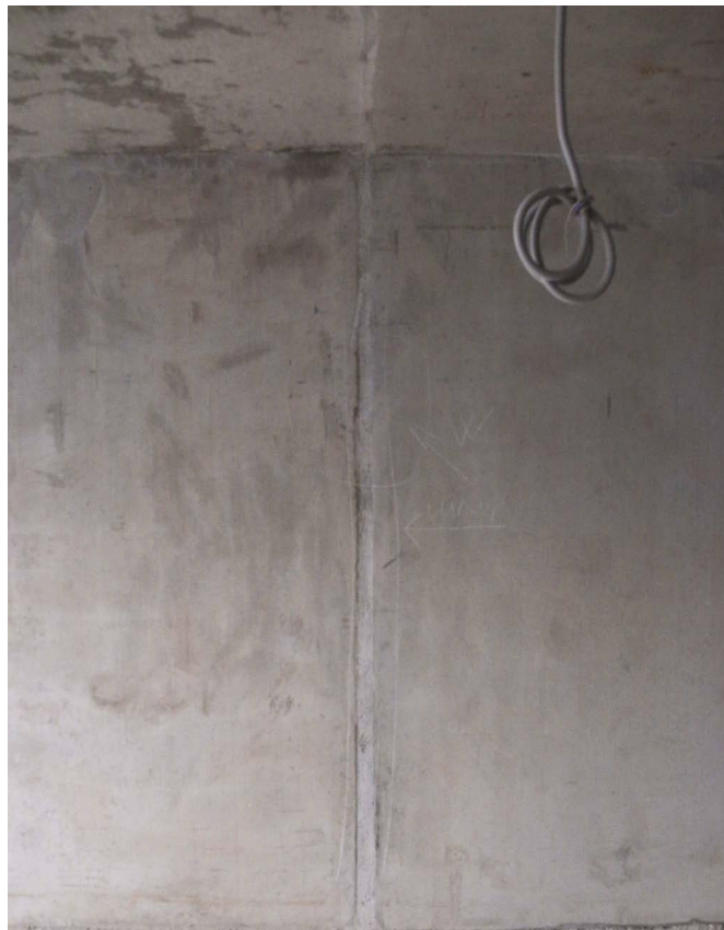
Figure 24. Finished wall joint.
