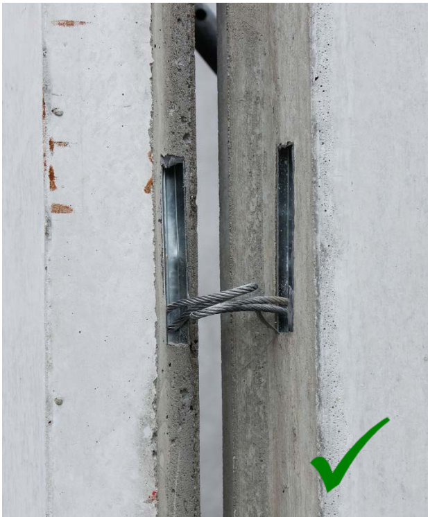
Position of wire loops before placement of the longitudinal rebar
