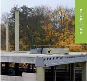
Downstands are included to Deltabeams to support pre-stressed hollow-core and filigran slabs in different elevations. Composite beams are integrated into the slab. The composite columns of the upper floor are attached to the Peikko anchor bolts of the composite columns on the ground floor.
