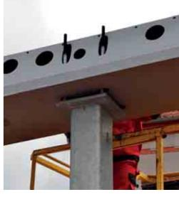
The perfect match of the connections means that the prefabricated Deltabeams can be installed in a short amount of time on composite columns that can bear loads already in assembly state.
