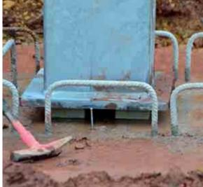
Composite Columns by Peikko are available as prefabricated products with the necessary connections and can be erected, assembled and aligned without temporary bracing.
