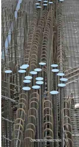
"When we speak about big spans and heavy loaded concrete elements, the use of forged heads as anchorage of reinforcement can be the best technically feasible and cost efficient solution," **Gatis Pocs**, product manager of punching reinforcement at Peikko Group, said.
