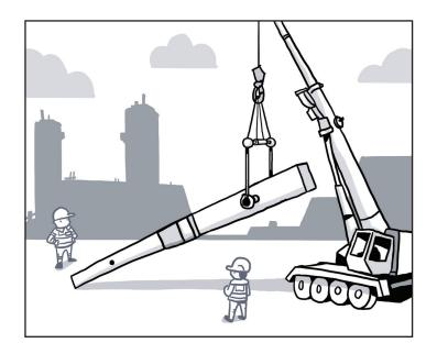
COMPATIBLE ANCHORS for tilting up a column
