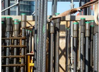
**MODIX®** Rebar Coupler Systems are CE marked
