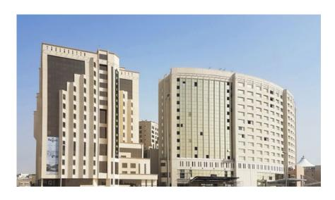
Al Rashid hotel and residential complex is located right next to Al Rashed Mall in Al Khobar. The complex is connect-ed to the mall by a bridge. Complex has a hotel and five residential build-ings connected to each other from the upper floors. The whole frame of the building is designed with Peikko column connections with a remarkable amount of HPKM® column shoes and bolts. Most of the other connections are designed with welding plate connections also manufactured by Peikko.
