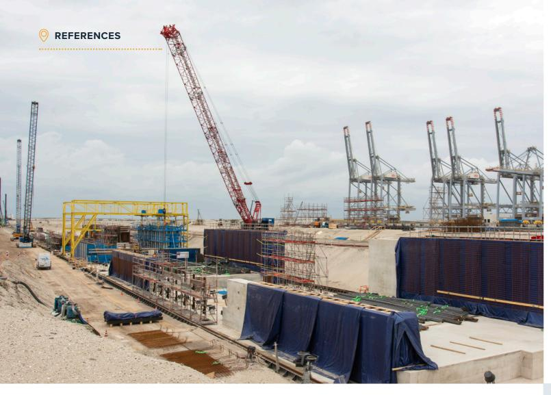
onstructed in 20 meter pieces, new quay walls are huge, U-shaped and cast in situ structures with a lot of reinforcement.
