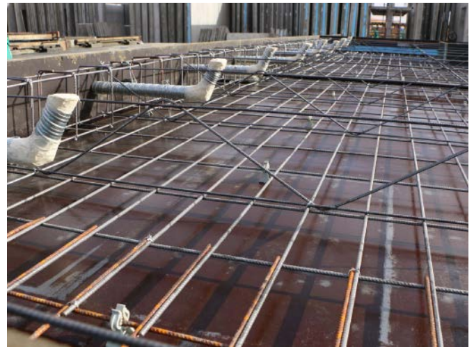
Figure 19. Diagonal ties installation with mesh.
