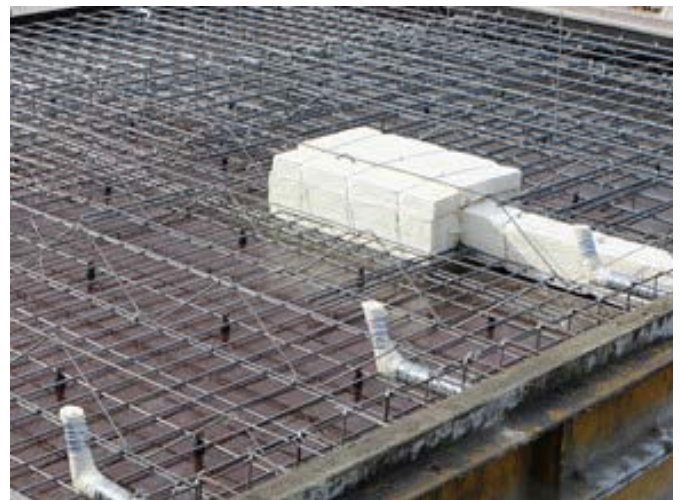
Figure 20. PD ties after installation of insulation.
