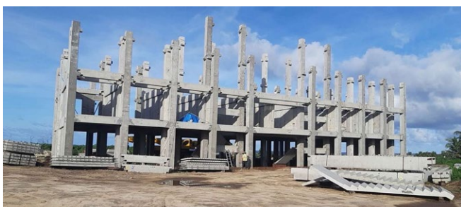
FIGURE 28 PHOTO OF CONSTRUCTION SITE WITH PRECAST STRUCTURAL ELEMENTS INSTALLATION IN PROGRESS
