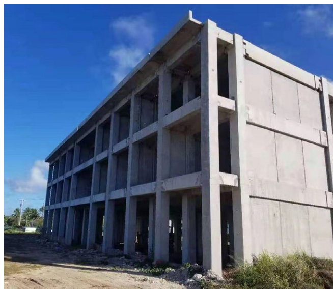
FIGURE 29 PHOTO OF CONSTRUCTION SITE WITH COMPLETED STRUCTURAL ELEMENTS INSTALLATION
