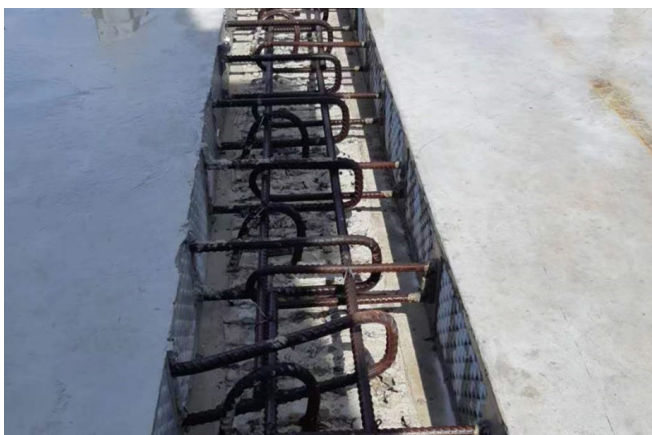
FIGURE 27 PHOTO OF JOINT ALONG PRECAST SLAB UNITS
