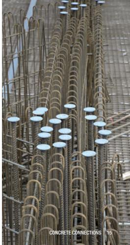
"When we speak about big spans and heavy loaded concrete elements, the use of forged heads as anchorage of reinforcement can be the best technically feasible and cost efficient solution," **Gatis Pocs**, product manager of punching reinforcement at Peikko Group, said.
