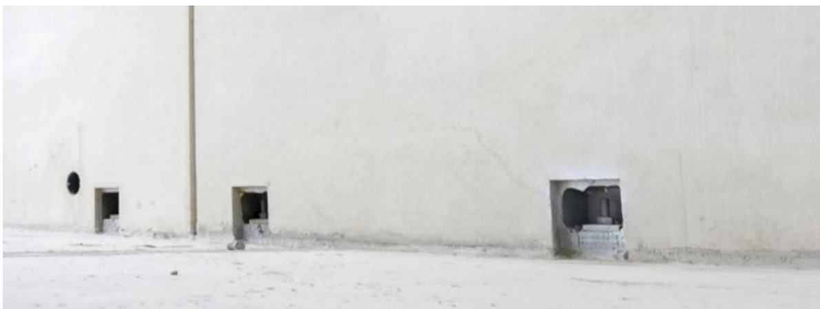
Fig. 3 The wall connections installed
