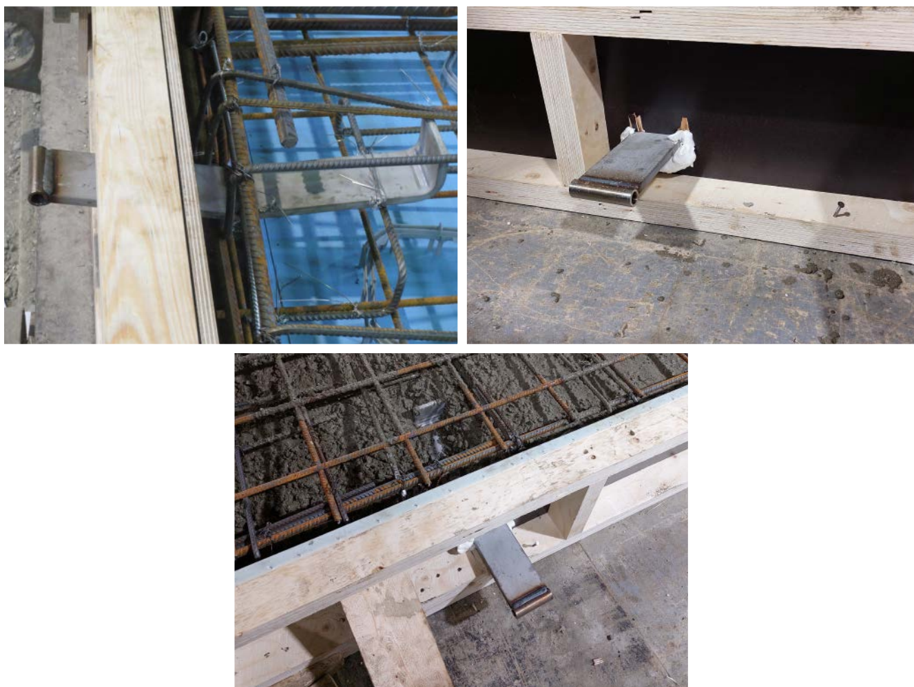
Figure 12. Installation of the PS Balcony Slab Connector Part B to wooden formwork.
