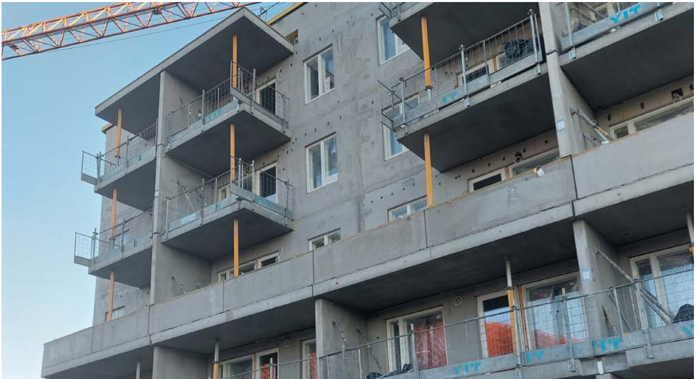
Figure 1. Divided balcony slabs.
