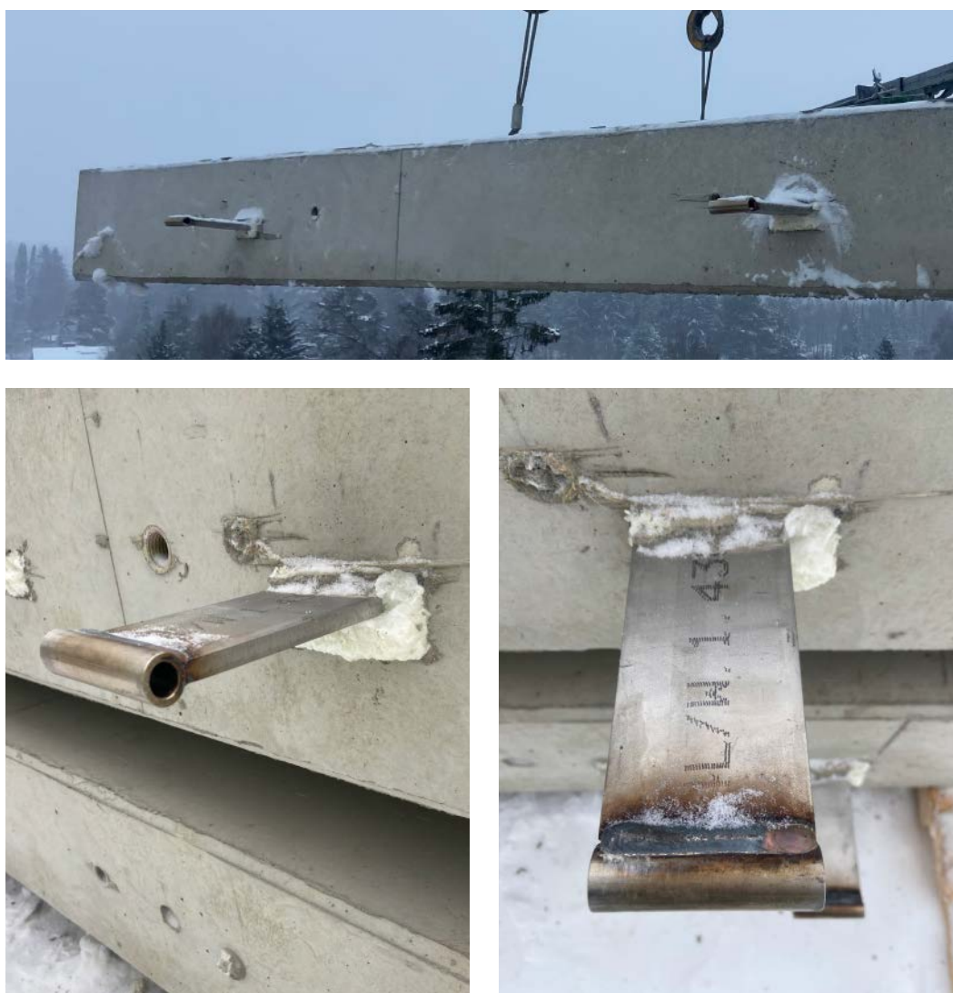
Figure 16. Balcony slab with PS Part B.
