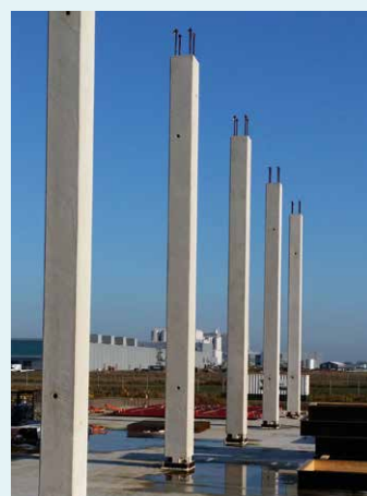
FIGURE 1. (A) PEIKKO'S BOLTED COLUMN-TO-FOUNDATION CONNECTION (ADAPTED FROM [16], [17])
