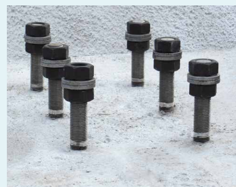
FIGURE 1. (A) PEIKKO'S BOLTED COLUMN-TO-FOUNDATION CONNECTION (ADAPTED FROM [16], [17])
