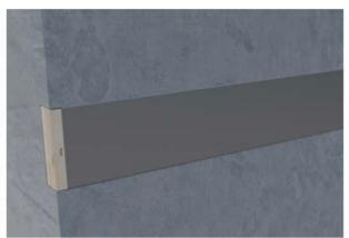
Remove the ARBOX® steel cover by cutting the tapes that secure it. Then place the claw of a hammer at one end and pull it away to expose the pre-bent bars.
