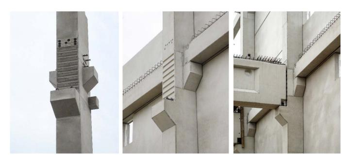
Connecting a COPRA® Anchoring Coupler with a BECO® Beam Shoe with the help of a threaded bar step by step.
