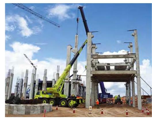
topping, which was 500 mm in depth, with the precast columns.
