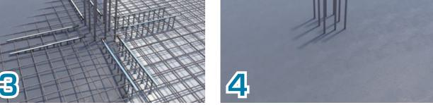
• Bottom installation: DSA Rail is placed below the main reinforcement of the slab prior to the installation of the bending reinforcement. In order to achieve a sufficient concrete cover of the headed studs, plastic spacers are mounted to the DSA Rail. Spacers are ordered separately.
