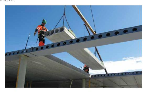
Floor units should be assembled directly on the beam ledge. Usage of neoprene is not recommended. Floor units should be assembled so that there is a gap of a maximum of 30 mm between the DELTABEAM's web and the end of the floor unit. If this gap is exceeded, contact Peikko or the structural engineer. Finally, all holes on the bottom side of DELTABEAM (locations of consoles, Side connections and Gerber connections) should be blocked. The joint and ring reinforcement are also assembled.
